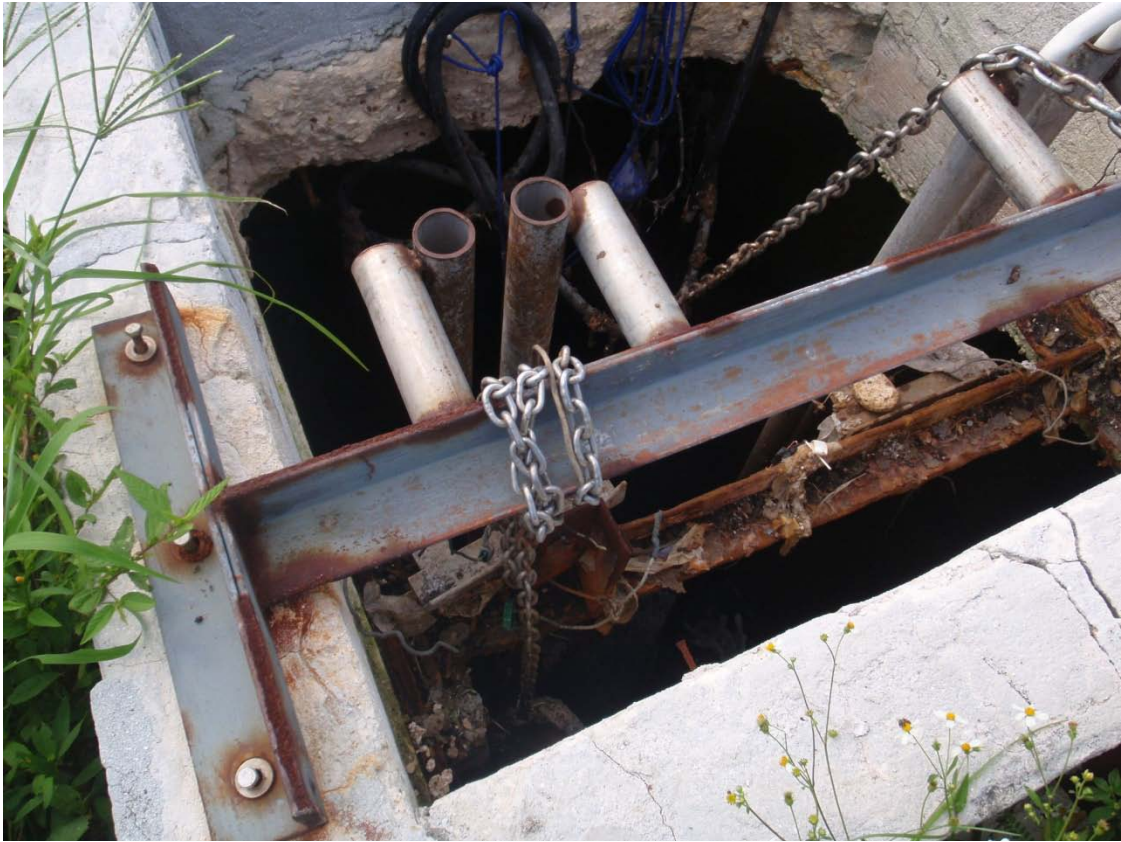
Figure 7: Fox Hill Wastewater Treatment Plant
