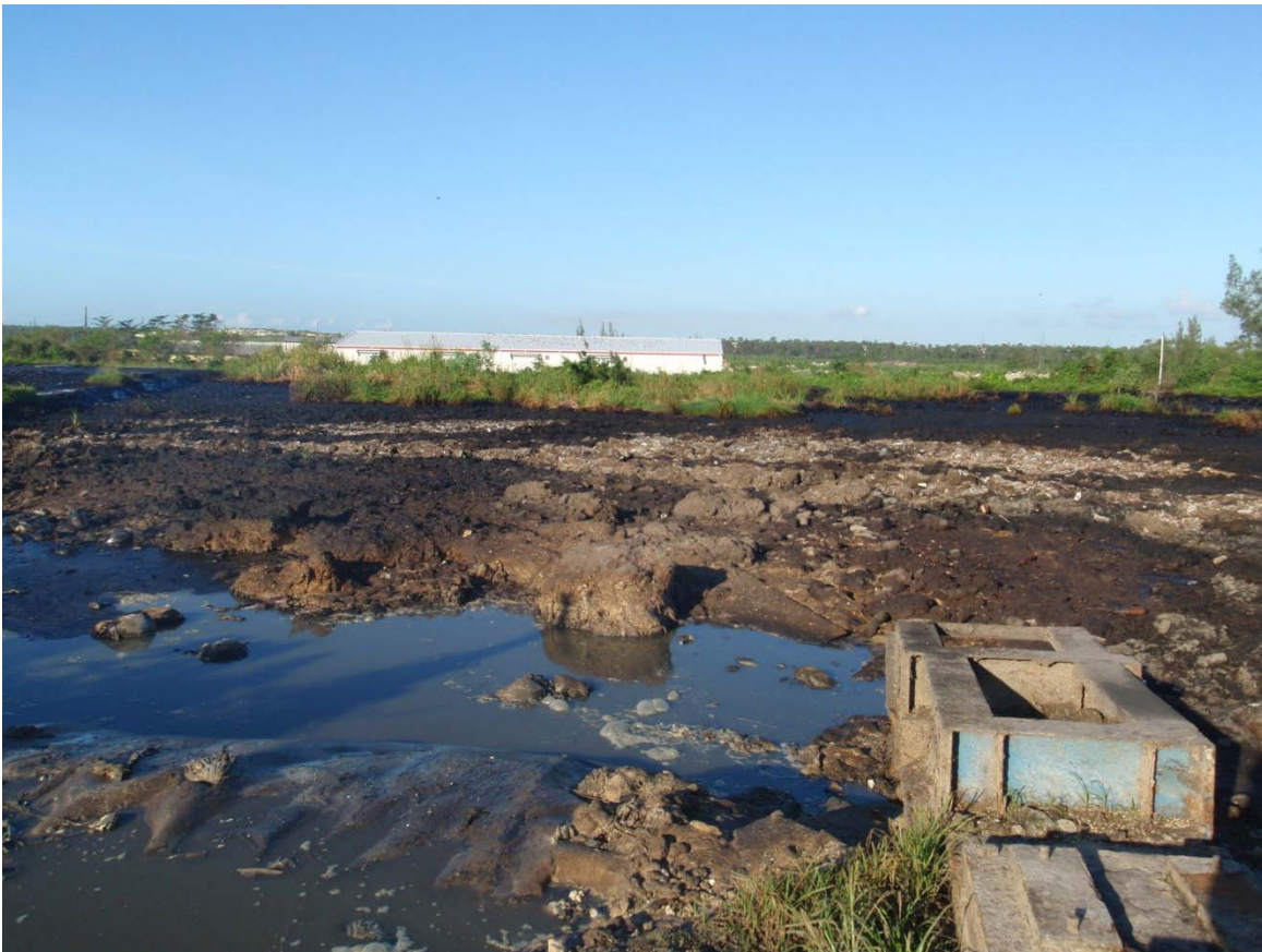
Figure 11: Lagoons at Septage and Sludge Facility
