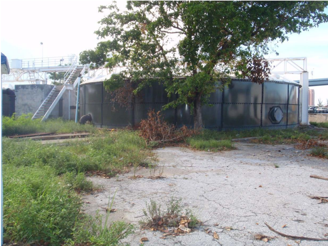
Figure 8: Malcolm Park Wastewater Treatment Plant – Storage Tanks
