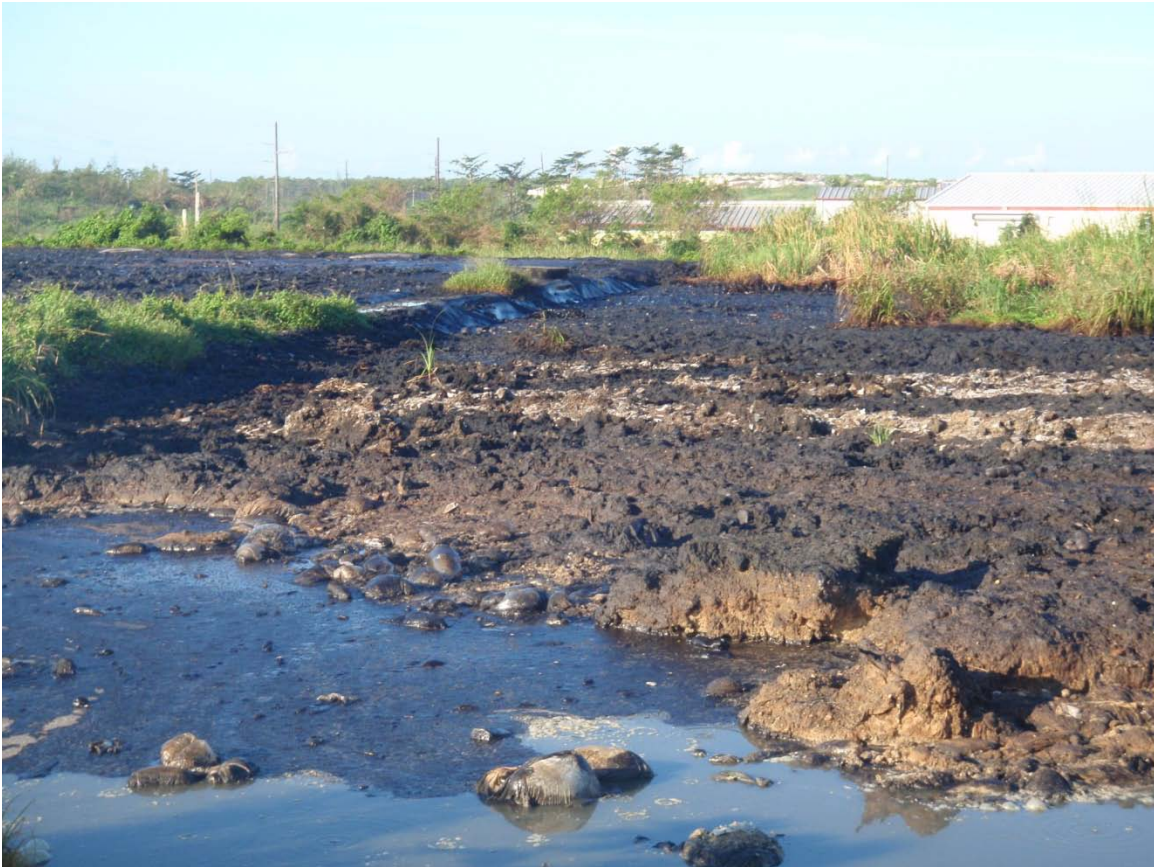
Figure 12: Lagoons at Septage and Sludge Facility
